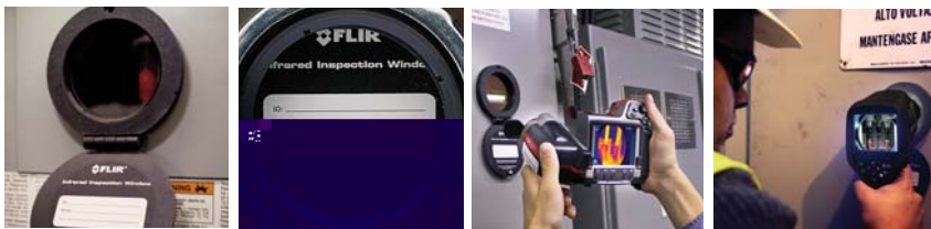
Hinged cover stays attached Window labeling/ID # Mount on Steel or Lexan Perform visual & Thermal inspections
